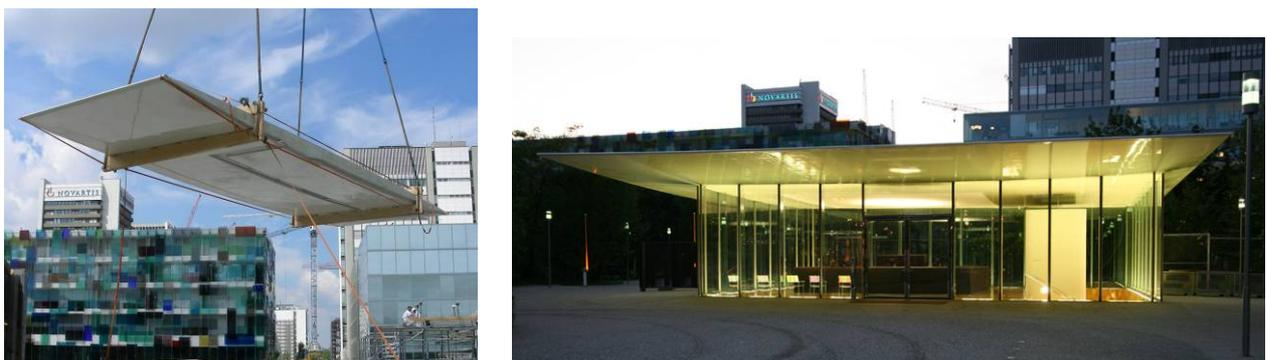
Fig. 1. Prefabricated multifunctional GFRP sandwich roof of Novartis Campus Main Entrance Building, (Keller et al. 2008)
